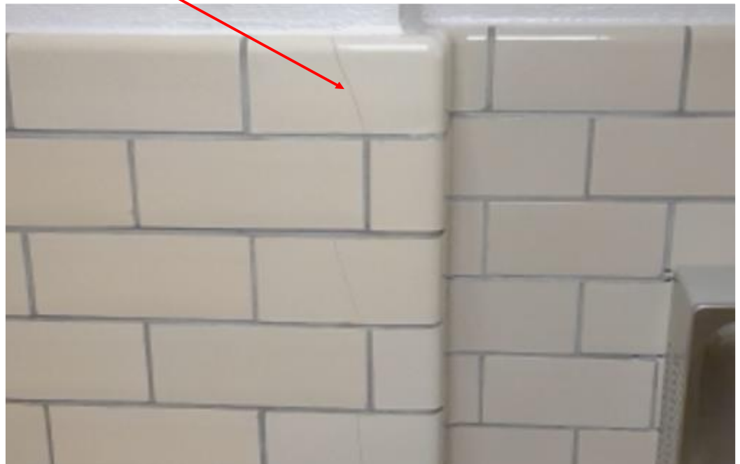
Existing crack in wainscoting
