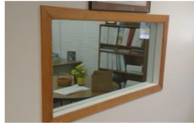
Existing non-compliant glazing
