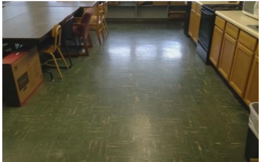
Existing asbestos containing floor tile
