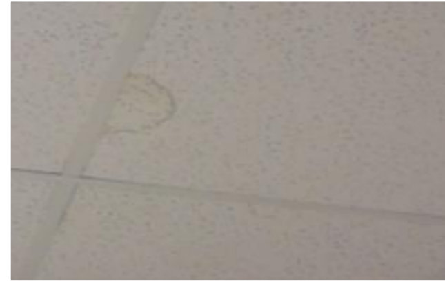
Existing water damaged ceiling tile
