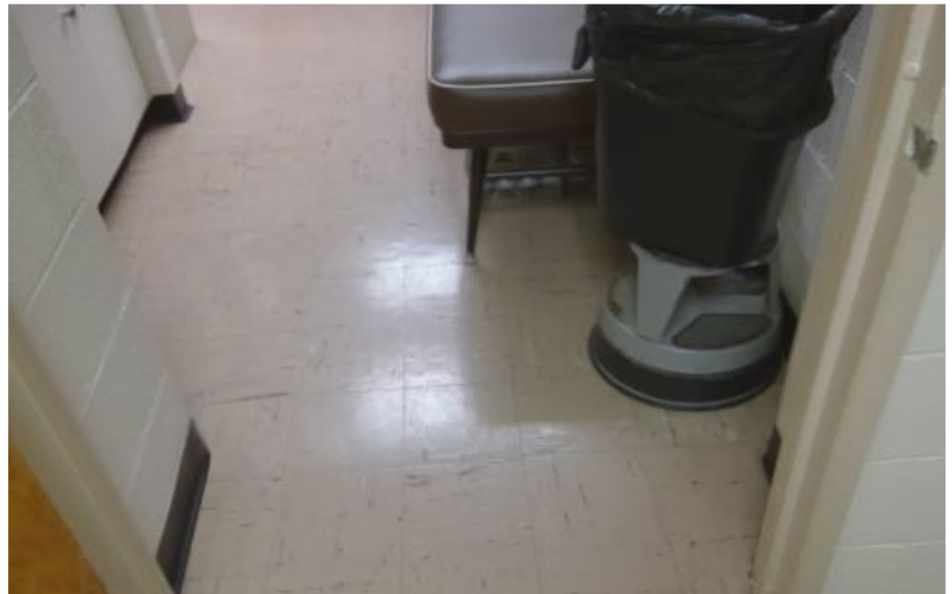
Existing asbestos containing floor tile
