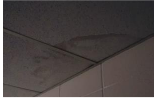
Existing water damaged ceiling tile
