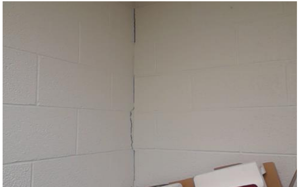
Existing masonry caulk joint
