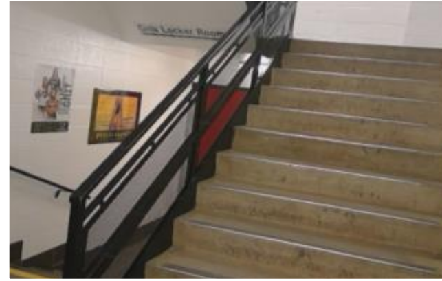
Existing non-compliant stair railings
