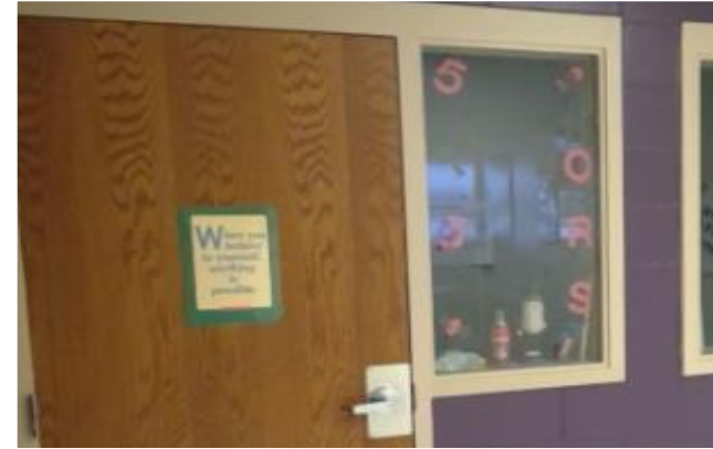
Existing non-compliant glazing
