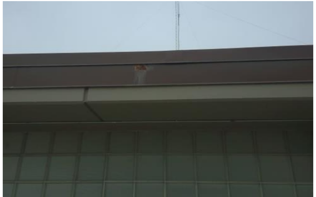
Existing damaged fascia
