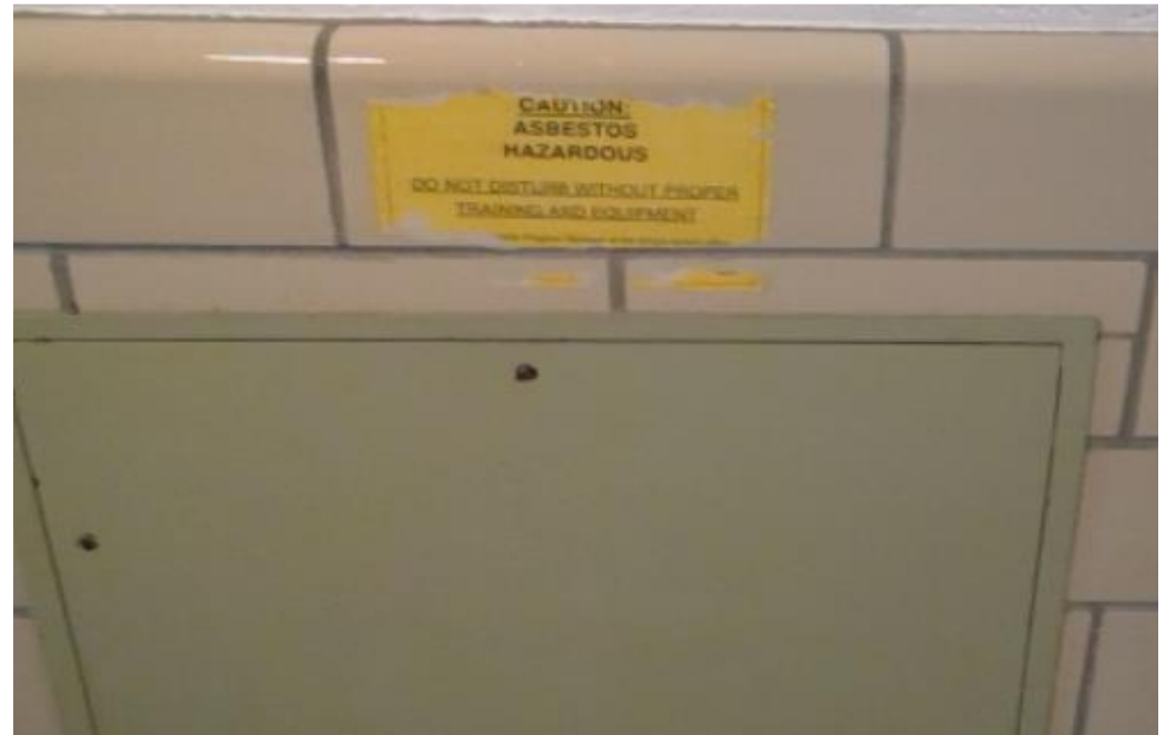
Asbestos insulation warning label
