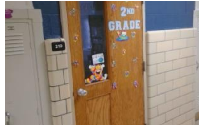
Existing non-compliant door and hardware
