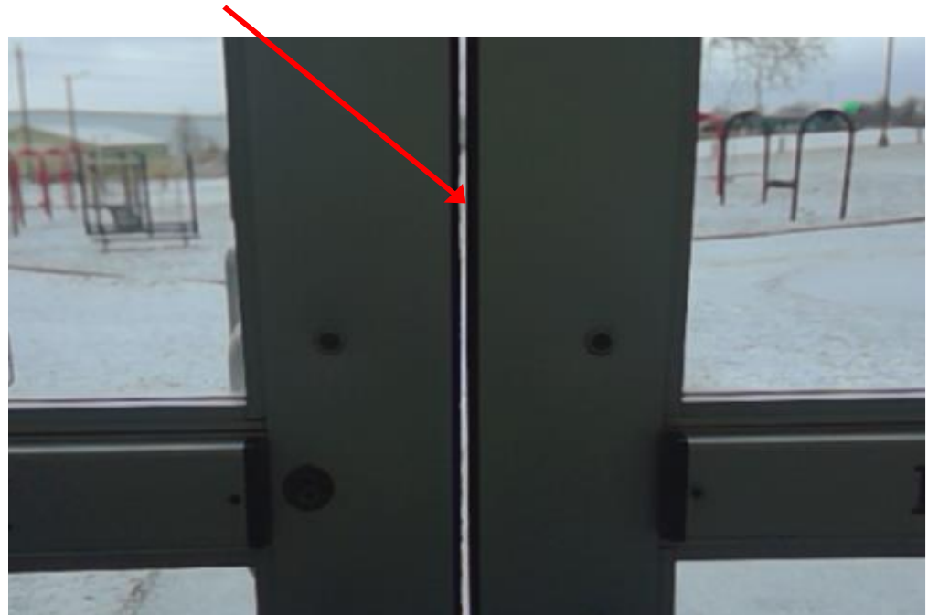
Existing air gap at exterior doors
