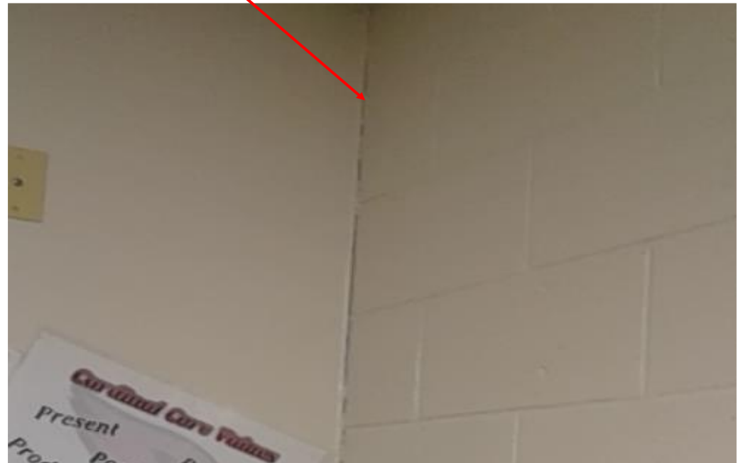
Existing masonry caulk joint
