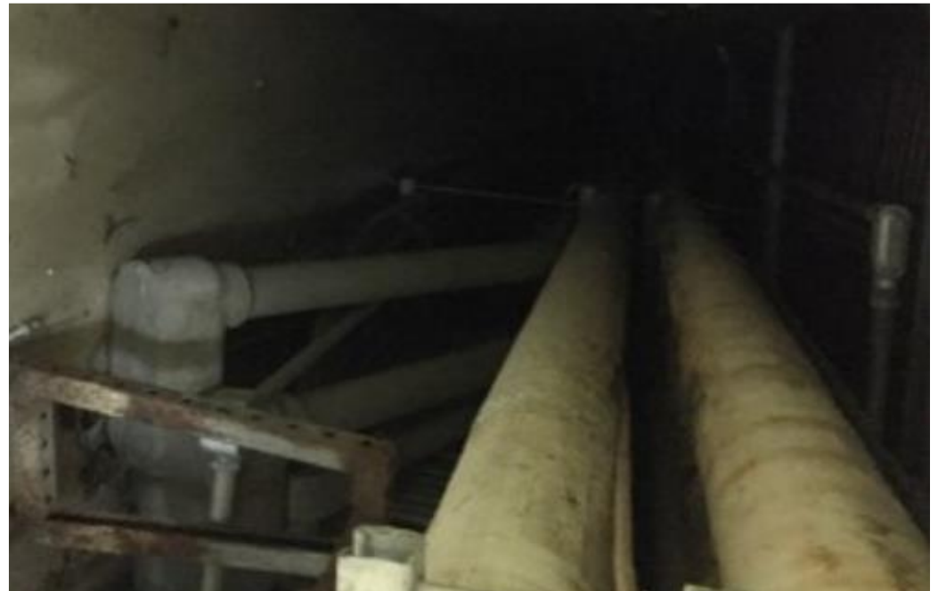
Existing asbestos insulation
