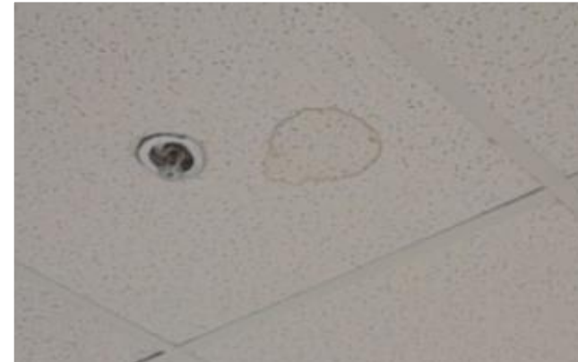
Existing water damaged ceiling tile
